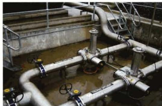
■ This New South Wales, Australia, irrigation project utilizes four off bersonInLine 7500 units and a small jacking InLine 250 system.
